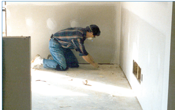
Use a razor knife, pole scraper, ect. to properly clean slab of mud, dry wall compound, paint etc.
